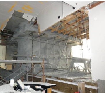
Overall View of Repair Using Shotcrete
